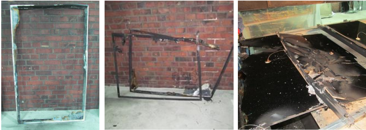
Figure 3-3: Damage from stress with 150 kW burner output, left: c-Si, center: CIS (transversely placed), right: CdTe (transversely placed)
