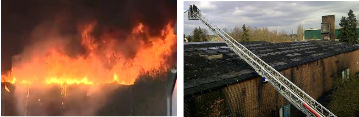
Figure 3-34: Electric arc event in a roof-mounted elevated PV system. Left: Bitumen roof sheeting burns with heavy smoke development and produces burning droplets. Right: Fortunately the building could be saved, photos: Goch Volunteer Fire Department
