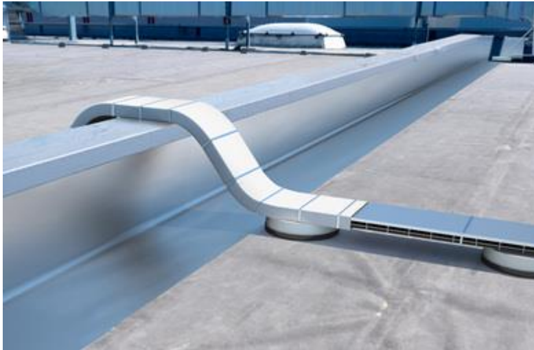
Figure 5-25: Fire protection bandages can prevent fire propagation across firewalls, photo: Obo Bettermann. [73]
