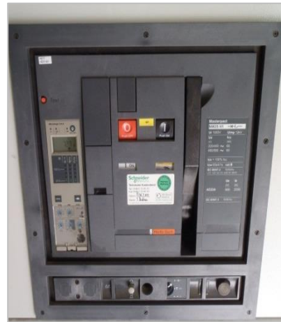
Figure 5-40: Load-break switch
