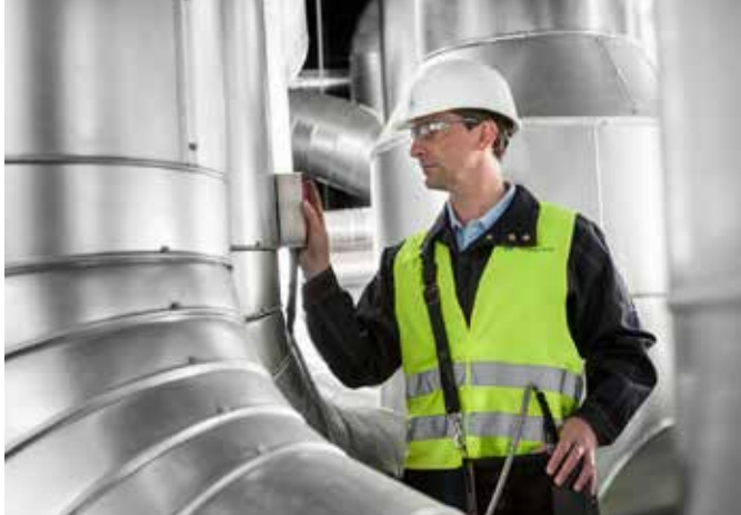
Inspection through insulation. Pulsed eddy-current inspection of a steel skirt through fire-proofing material.
